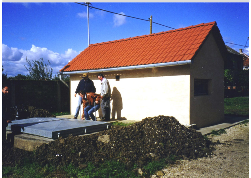
Vacuum Station at Csorna
