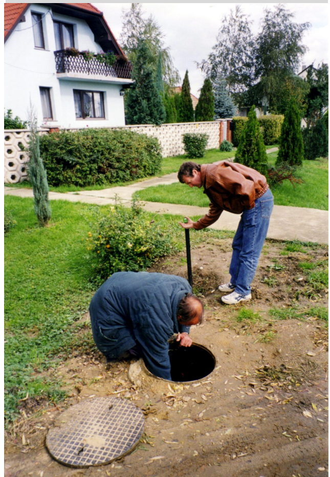
Valve Chamber Inspection
