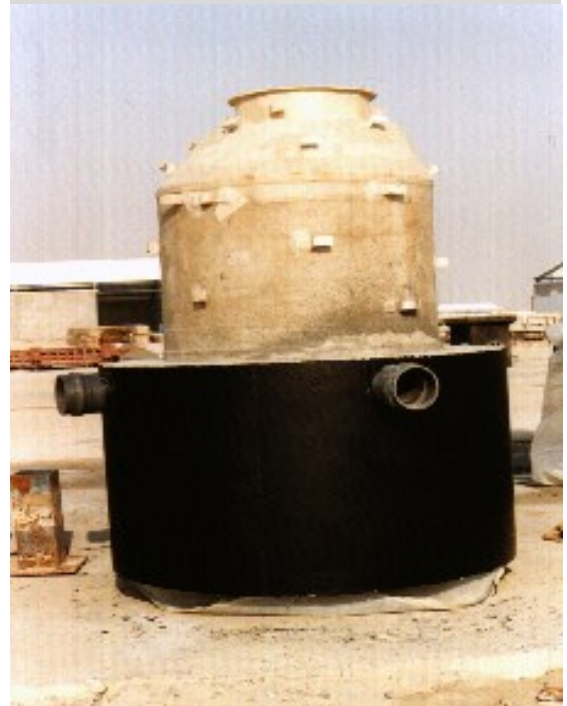
GRP Collection Sump with concrete anti-floatation collar
