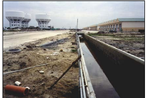
Deep Stormwater Drains
