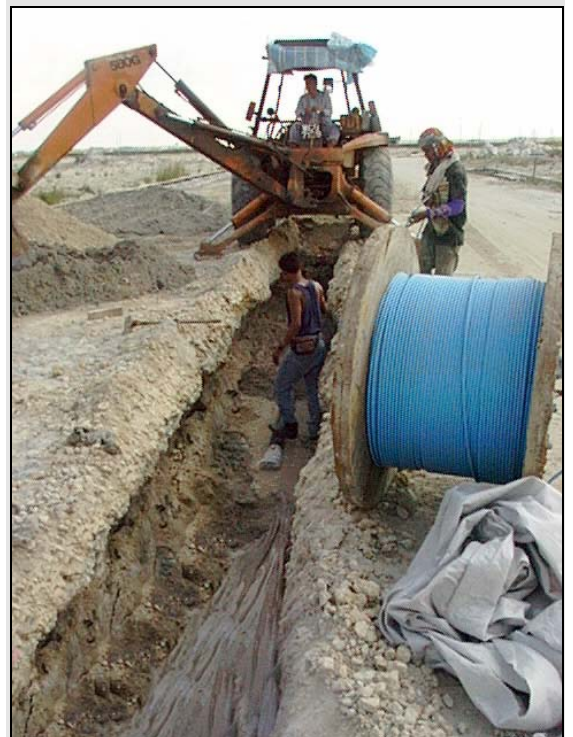
Cable Works and Trenching
